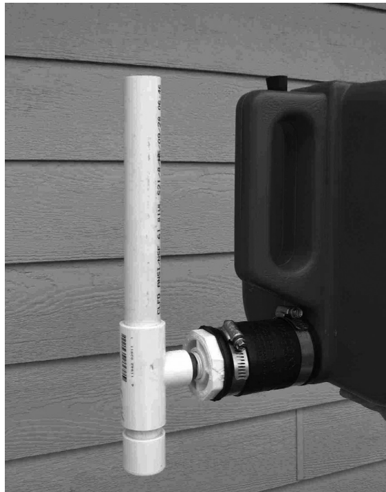
APPENDIX FIGURE 5. Reducing bushing and nipple for standpipe.
